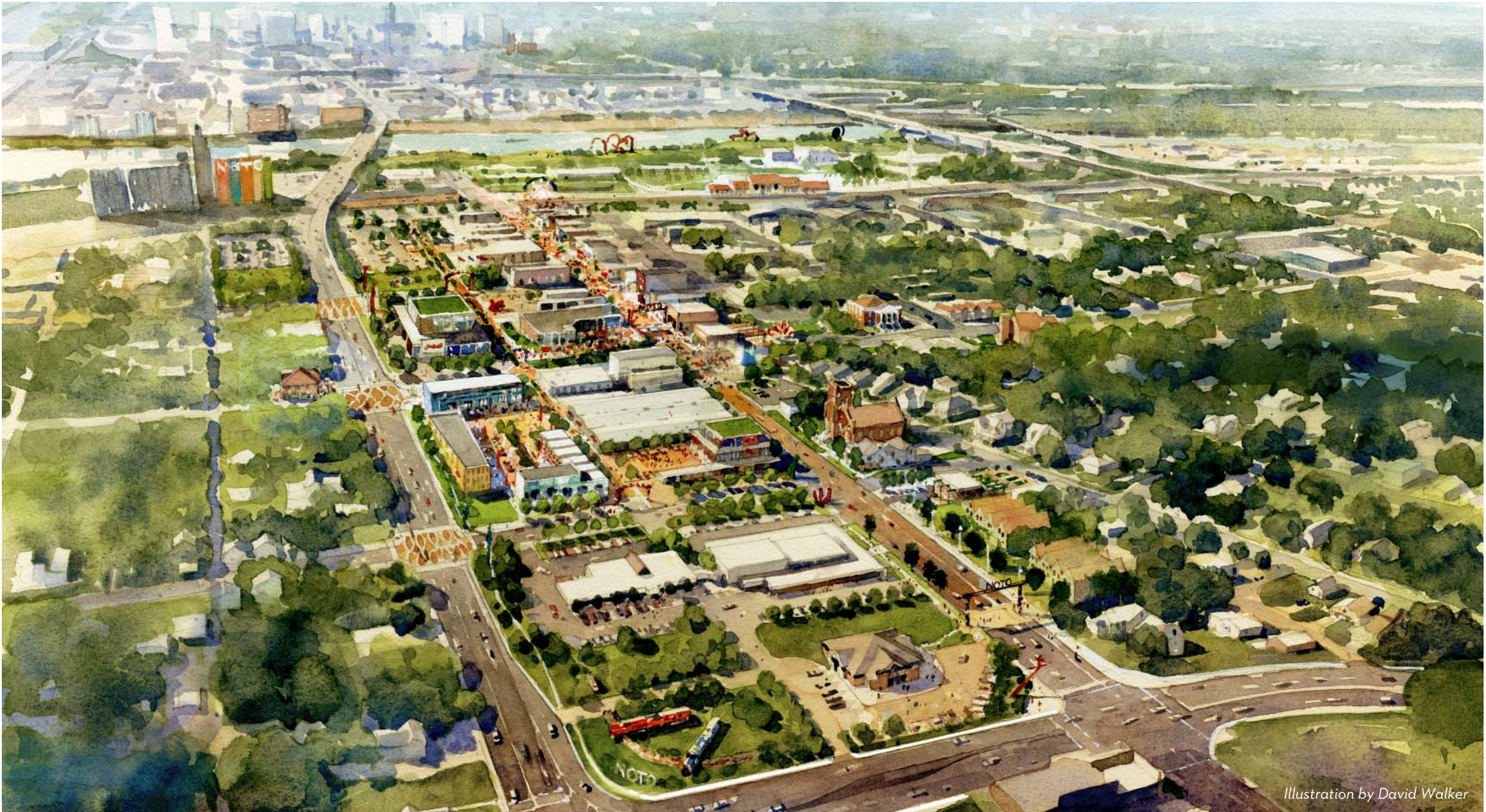
FIGURE 3.1 - DISTRICT VISION - LOOKING SOUTH FROM MORSE STREET - AERIAL VIEW
