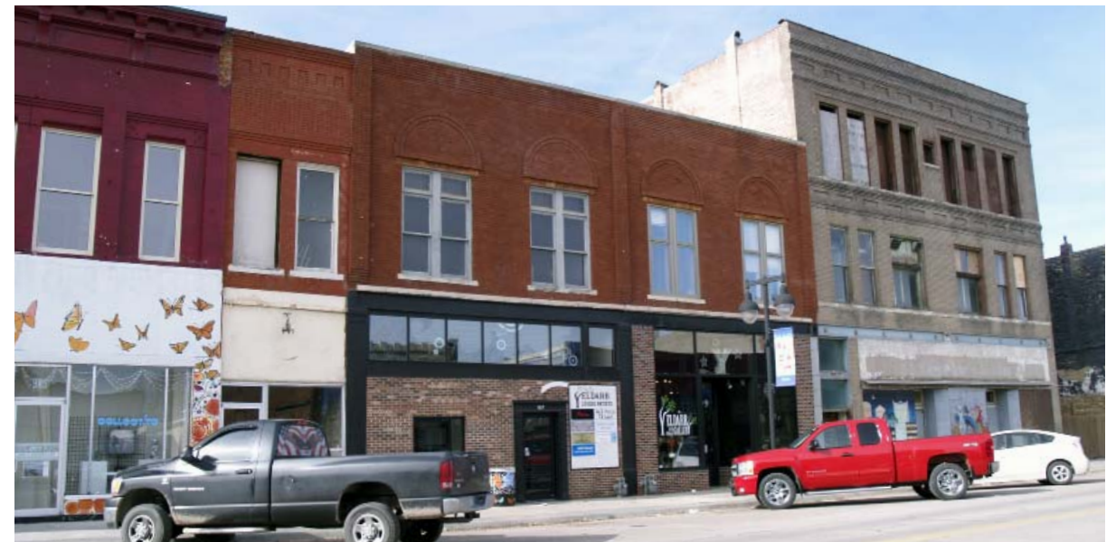
District buildings in need of facade and storefront improvements
