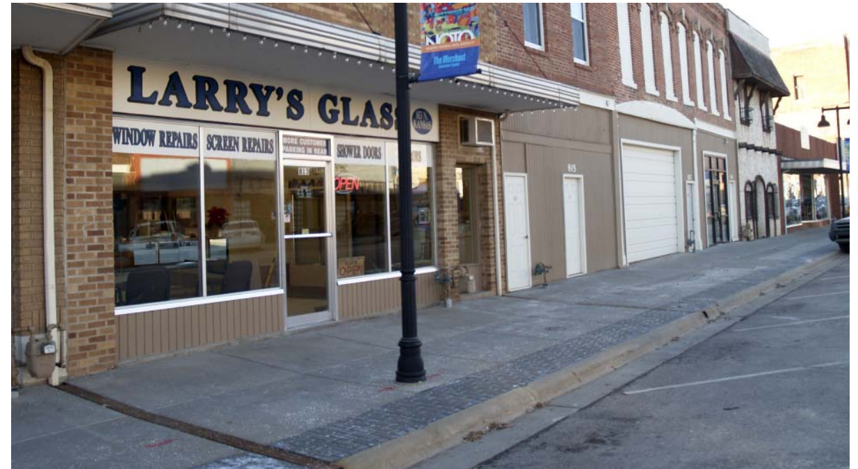
Streetscape conditions on Kansas Avenue
